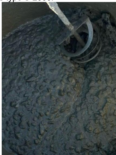
Fig. 1 - Preparing concrete by adding aggregate and cement
