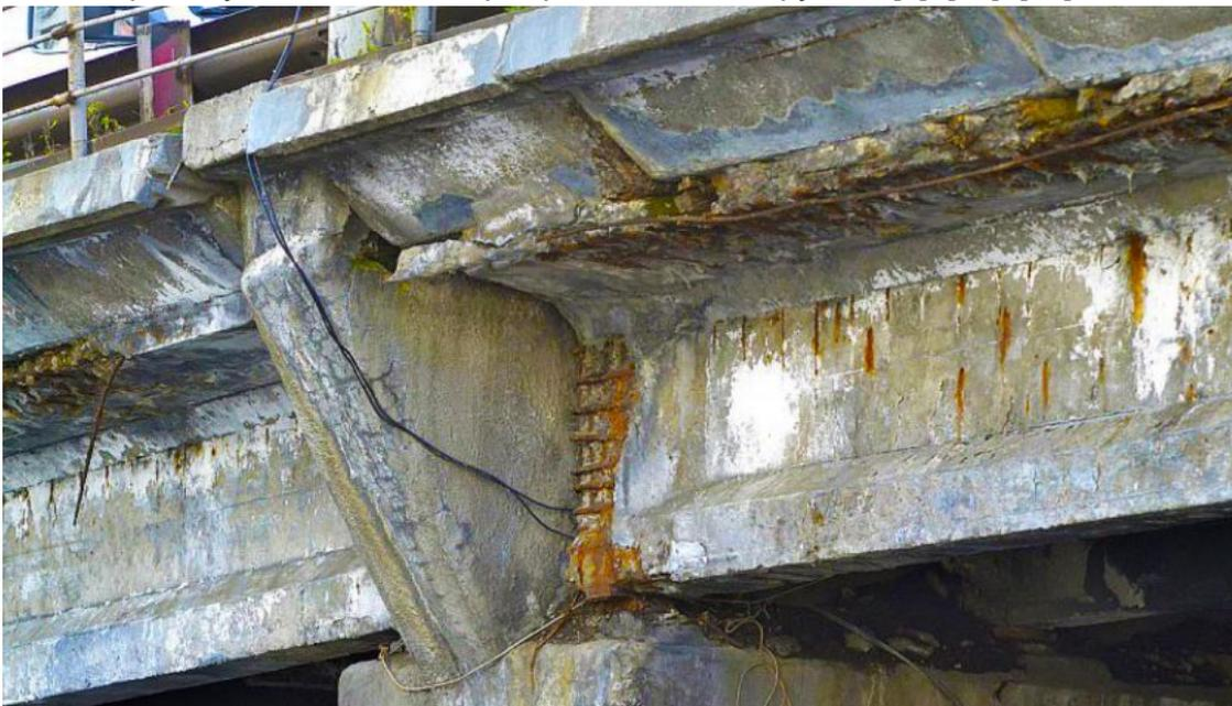
**Fig. 1 – Damage of reinforced concrete bridge structure as a result of rebar corrosion [7]**
