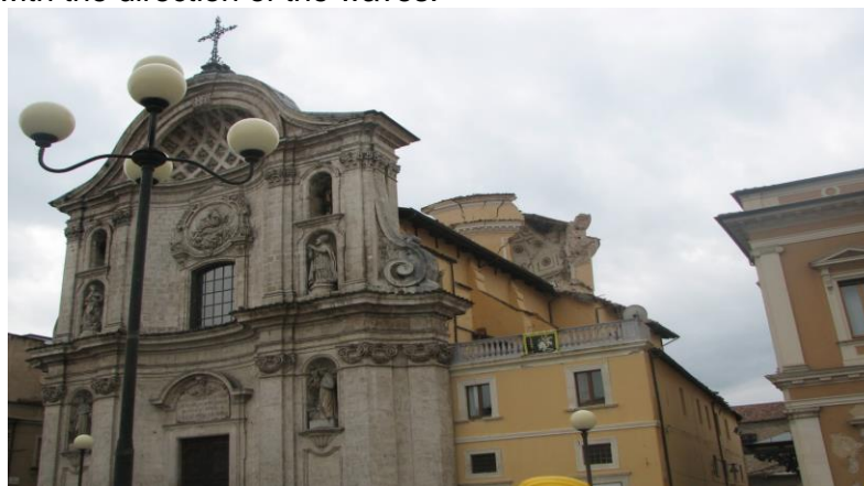
Fig. 8 - Church of Santa Maria del Suffraggio in Aquila, damaged after the seismic impact of the earthquake in 2009. (Original photo made by one of the authors)
