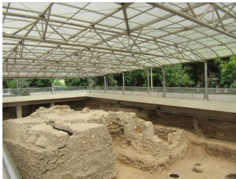
Fig. 9 Truss roof, near the Syntagma square in Athens, Greece (By authors)
