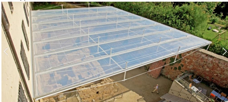
Fig. 6 Roof over the ruins behind the house of Luther, Wittenberg, Germany [22]
